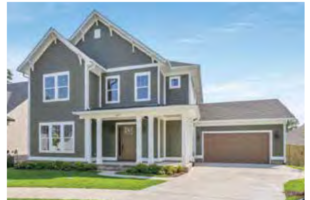
607 CHAMOMILE COURT, NICEVILLE, FL 4 Bedroom | 4 Bath | 3,048 SF $979,800 | construction completed Listed by Kelly Shephard 850.543.7353
