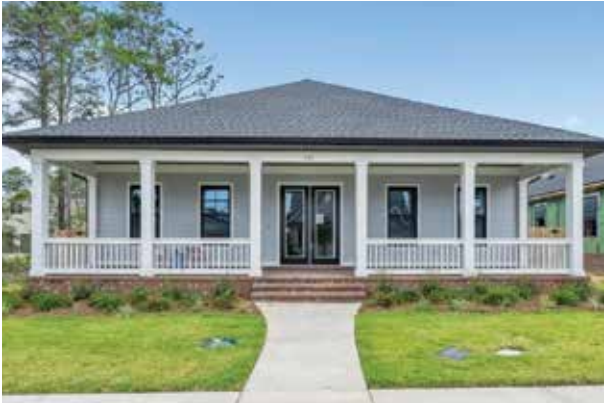
110 CARAWAY DRIVE, NICEVILLE, FL 4 Bedroom | 3 Bath | 2,481 SF $749,900 | construction completed Listed by Kelly Shephard 850.543.7353
