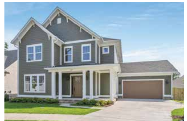
607 CHAMOMILE COURT, NICEVILLE, FL 4 Bedroom | 4 Bath | 3,048 SF $999,800 | construction completed Listed by Kelly Shephard 850.543.7353
