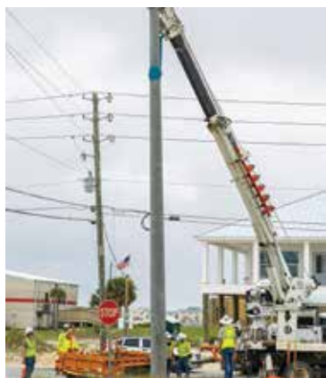
Crews install a concrete power pole in Northwest Florida to improve resiliency during hurricanes and severe weather and also enhance reliability during day-to-day conditions.
