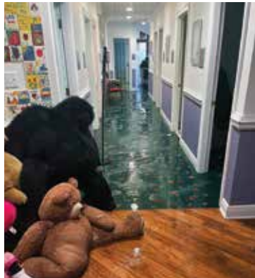
ECCAC's Niceville Center was severely damaged when their building's sprinkler system put out a fire that caused significant subsequent water damage.
